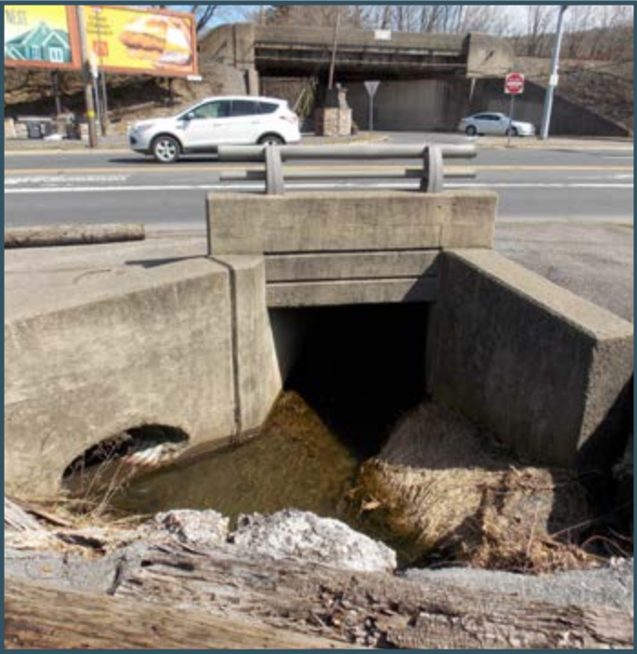
Culverts, such as those that run under State Avenue, should be routinely checked for debris.
