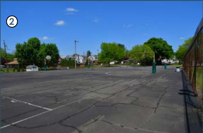
The existing basketball courts need to be resurfaced, and the fence should be replaced.
