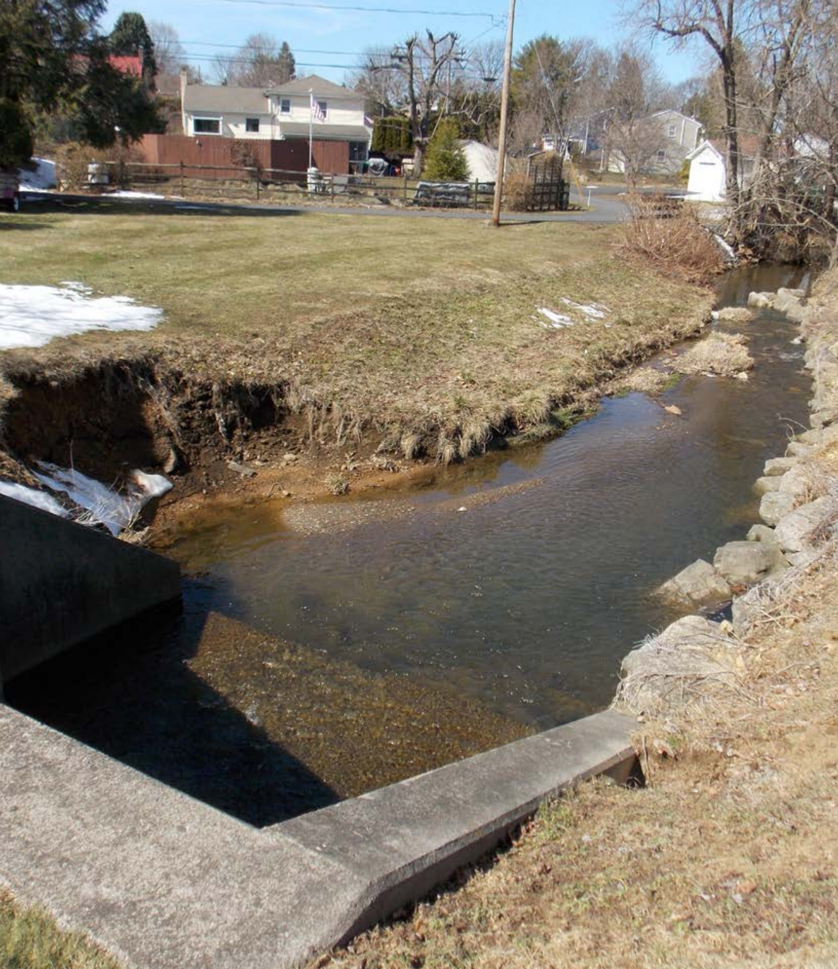
Streambank erosion along the unnamed tributary of Little Lehigh Creek on the north side of E. Harrison Street.
